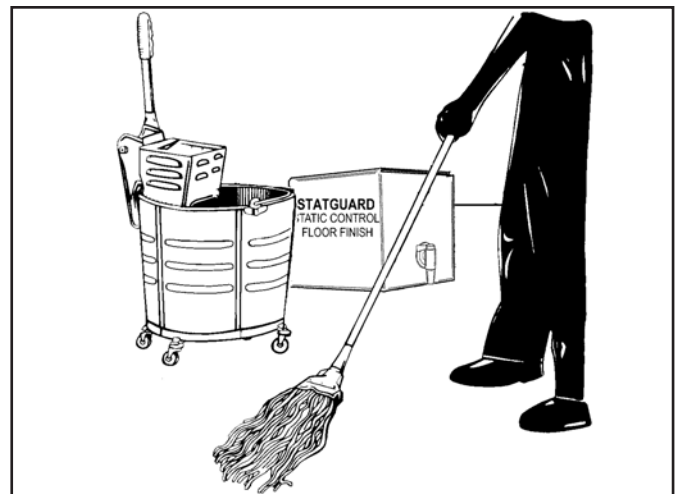
Figure 4. Applying floor finish.
